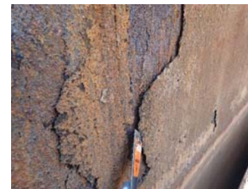
Fig.11 Corrosion on internal shell.
