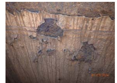
Fig.12 Corrosion on internal shell.
