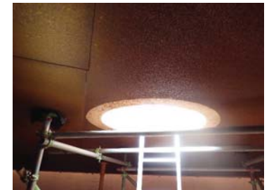
Fig.20 Surface corrosion on under roof deck.
