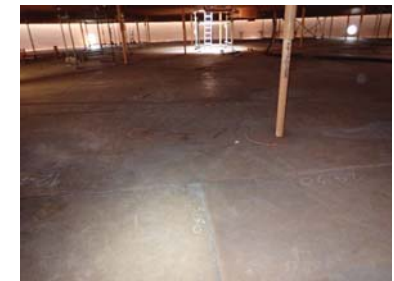
Fig.4 Normal condition on bottom plate.
