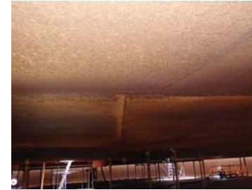
Fig.17 Surface corrosion on under roof deck.
