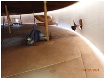
Fig.7 Normal condition on annular plate.
