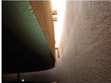
Fig.13 Corrosion on internal shell 0.5-2 mm depth (shell course 1).
