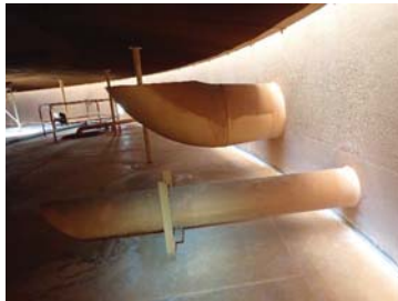
Fig.21 Normal condition on internal pipe.
