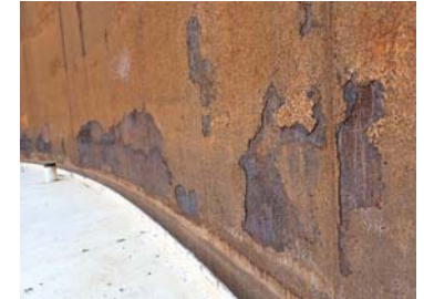
Fig.10 Corrosion on internal shell.
