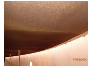
Fig.19 Surface corrosion on under roof deck.
