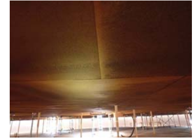
Fig.18 Surface corrosion on under roof deck.
