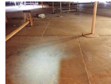
Fig.3 Normal condition on bottom plate.
