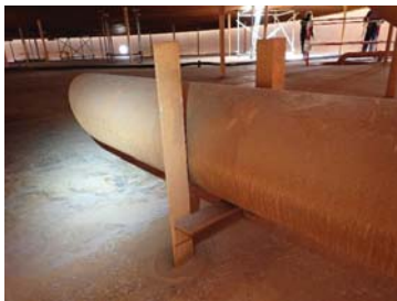
Fig.23 Normal condition on internal pipe.
